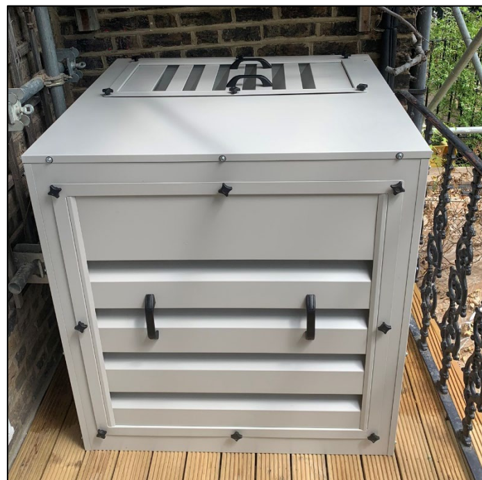
Condenser inside an Acoustic Louvre Enclosure
