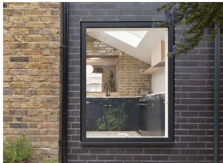
Example of a timber frame alu-clad triple glazed window with minimal sight-lines
