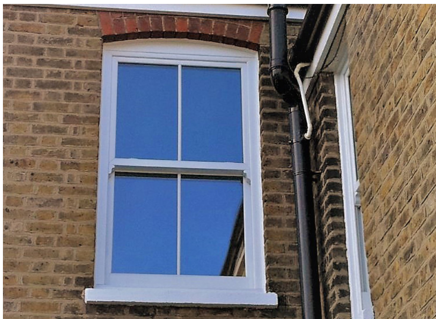
Example of traditional timber framed triple glazed sash window
