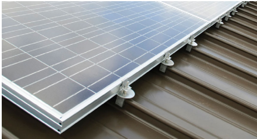
Example of S5 Clamp for fixing PV to standing seam roof
