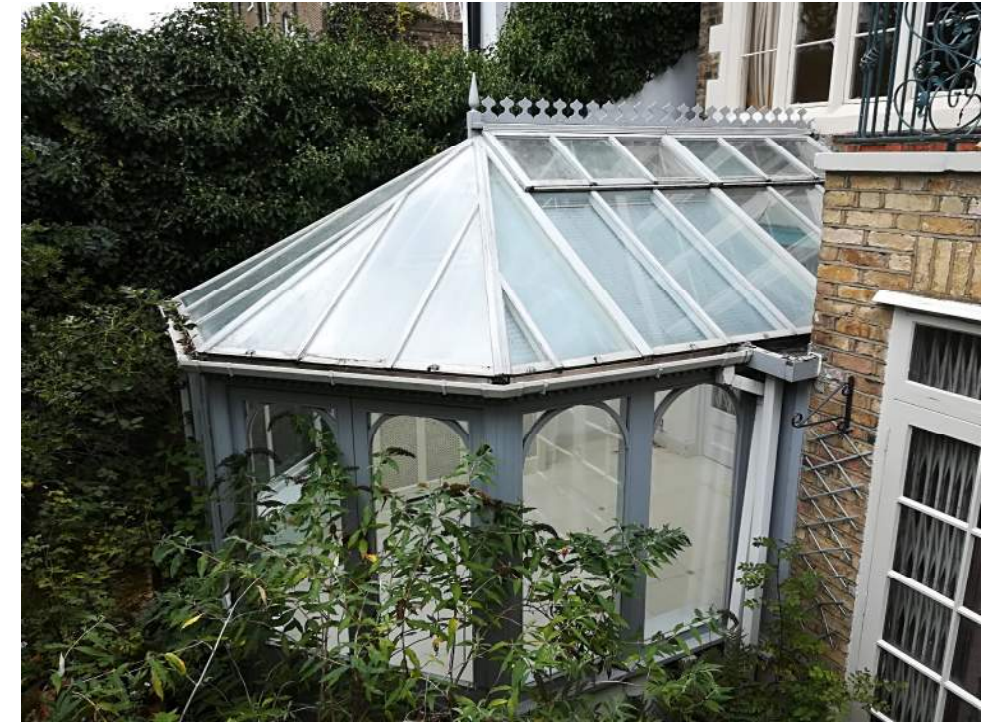
Figure 3.1 – Photo of existing conservatory
