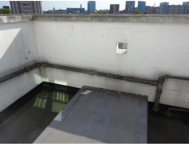
Proposal is to reduce window sill level to door threshold level by removing existing masonry wall outlined
