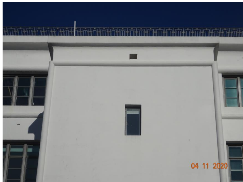
Fourth floor parapet wall
