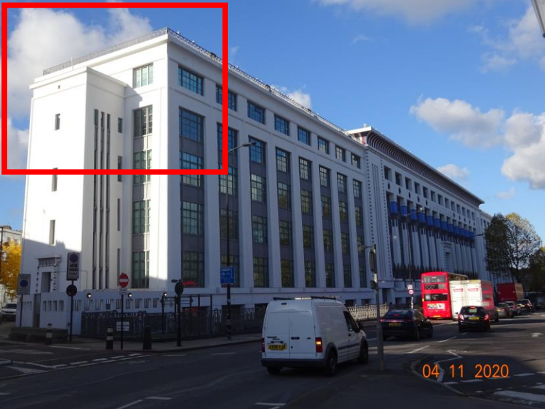
GLH looking north along Hampstead Road.
