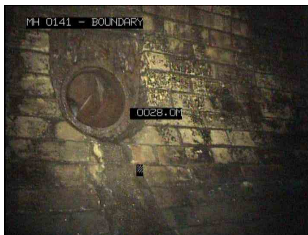
4, 00:04:48, 28.00 m Junction at 9 o'clock, diameter: 150mm
