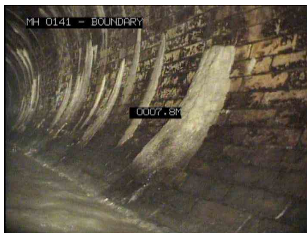
2, 00:01:46, 0.01 m Attached deposits, encrustation from 7 o'clock to 5 o'clock, 5% cross-sectional area loss, LIGHT PATCHES THROUGHOUT SEWER (SUGGESTS SLIGHT INFILTRATION SEEPAGE)
