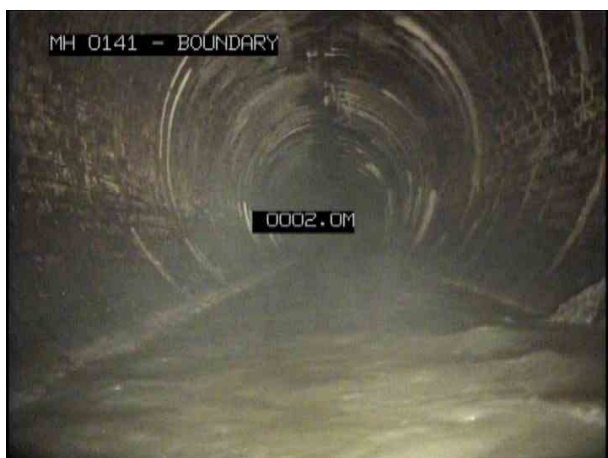
1, 00:00:25, 0.01 m Water level, 15% of the vertical dimension, FLOWING
