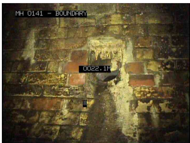
3, 00:03:36, 21.80 m Junction at 3 o'clock, diameter: 150mm
