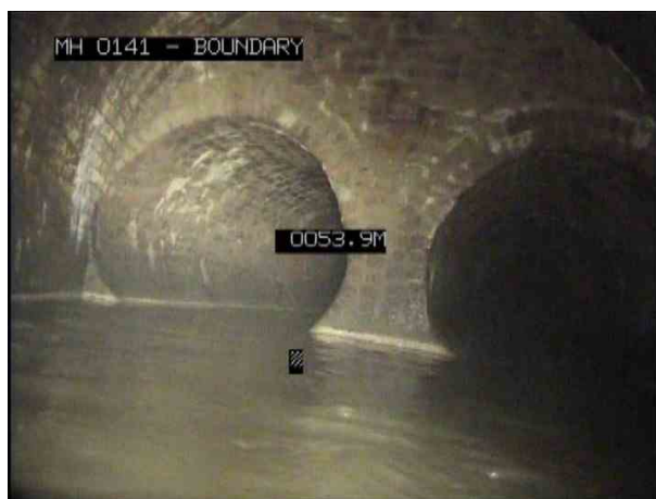
8, 00:08:06, 54.00 m General remark, PIPE OPEN UP & DIVERTS INTO DUEL SEWERS (APPROX. 1200MM DIA EACH)
