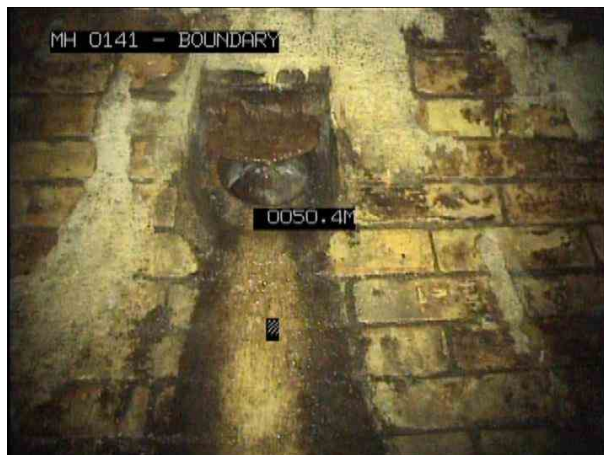
6, 00:06:48, 49.90 m Junction at 3 o'clock, diameter: 150mm
