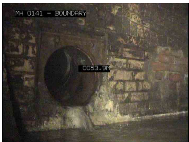
7, 00:07:45, 53.90 m Junction at 9 o'clock, diameter: 375mm
