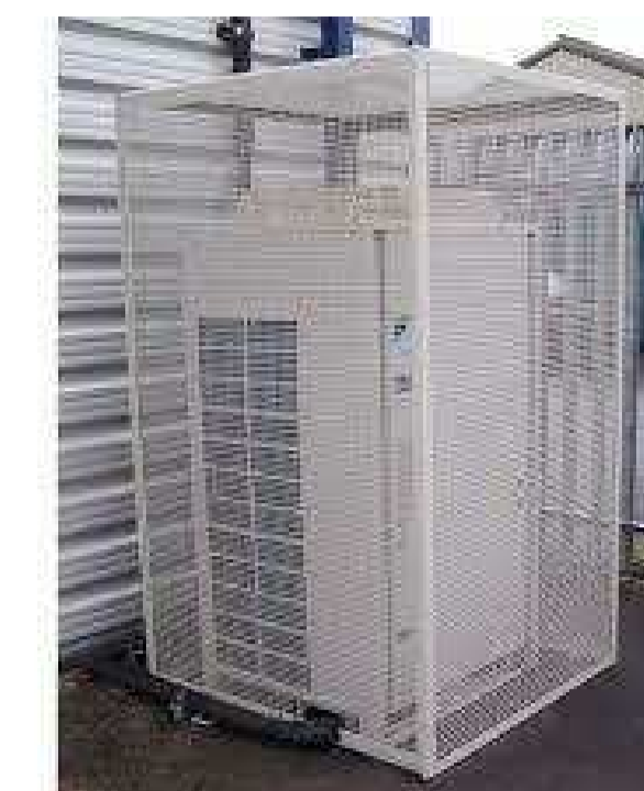
Typical Mechanical Plant Cage Example
