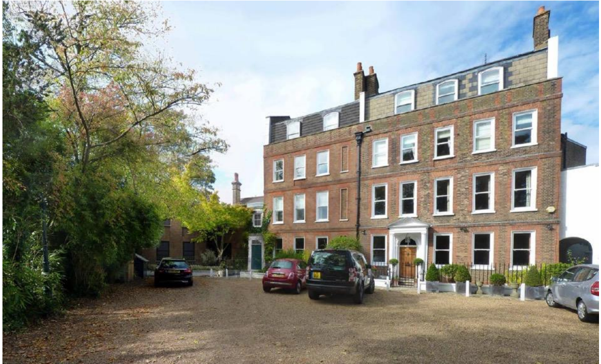
Photograph 1: Courtyard Parking Area
