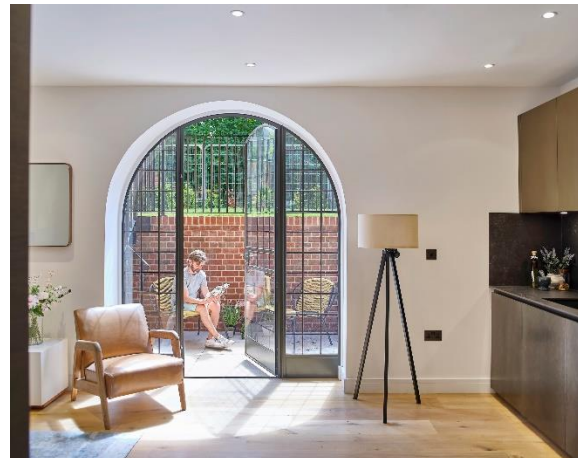
CRITTALL FRAMES USED IN THE FORMER APPLIANCE HALL (LEFT) AND LOWER GROUND FLOOR GARDEN ACCESS (RIGHT)
