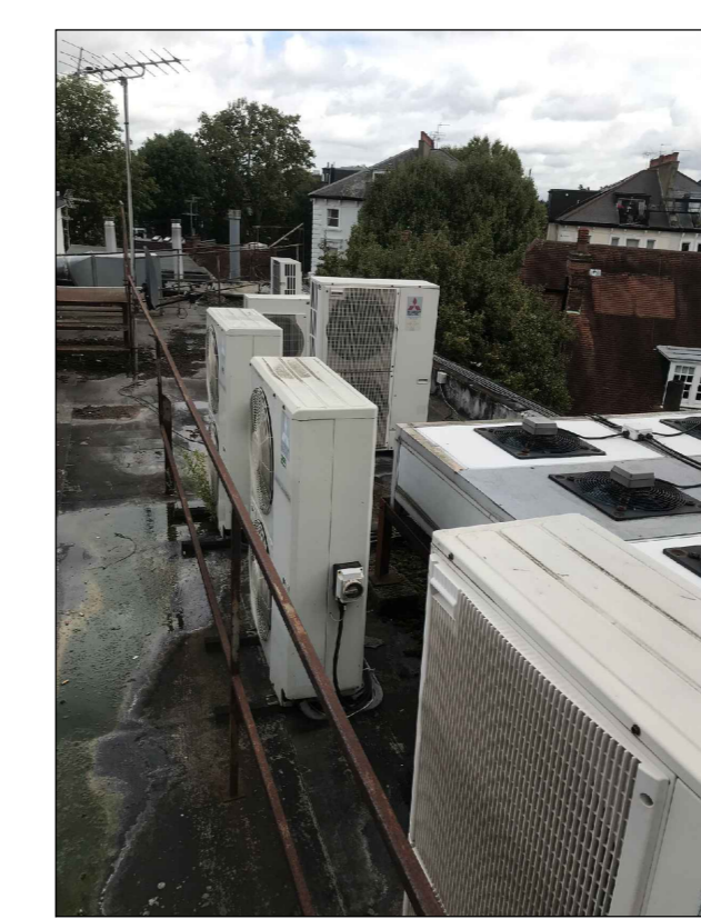
MITSUBISHI ?? CONDENSING UNIT ANTICIPATED SOUND PRESSURE LEVEL: 55dB(A) AT 1m DISTANCE/1.5m AFFL
