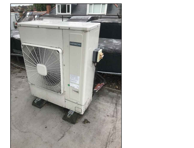
HITACHI RAS-4HANC1E CONDENSING UNIT ANTICIPATED SOUND PRESSURE LEVEL: 54dB(A) AT 1m DISTANCE/1.5m AFFL SOUND POWER LEVEL: 68dB(A)
