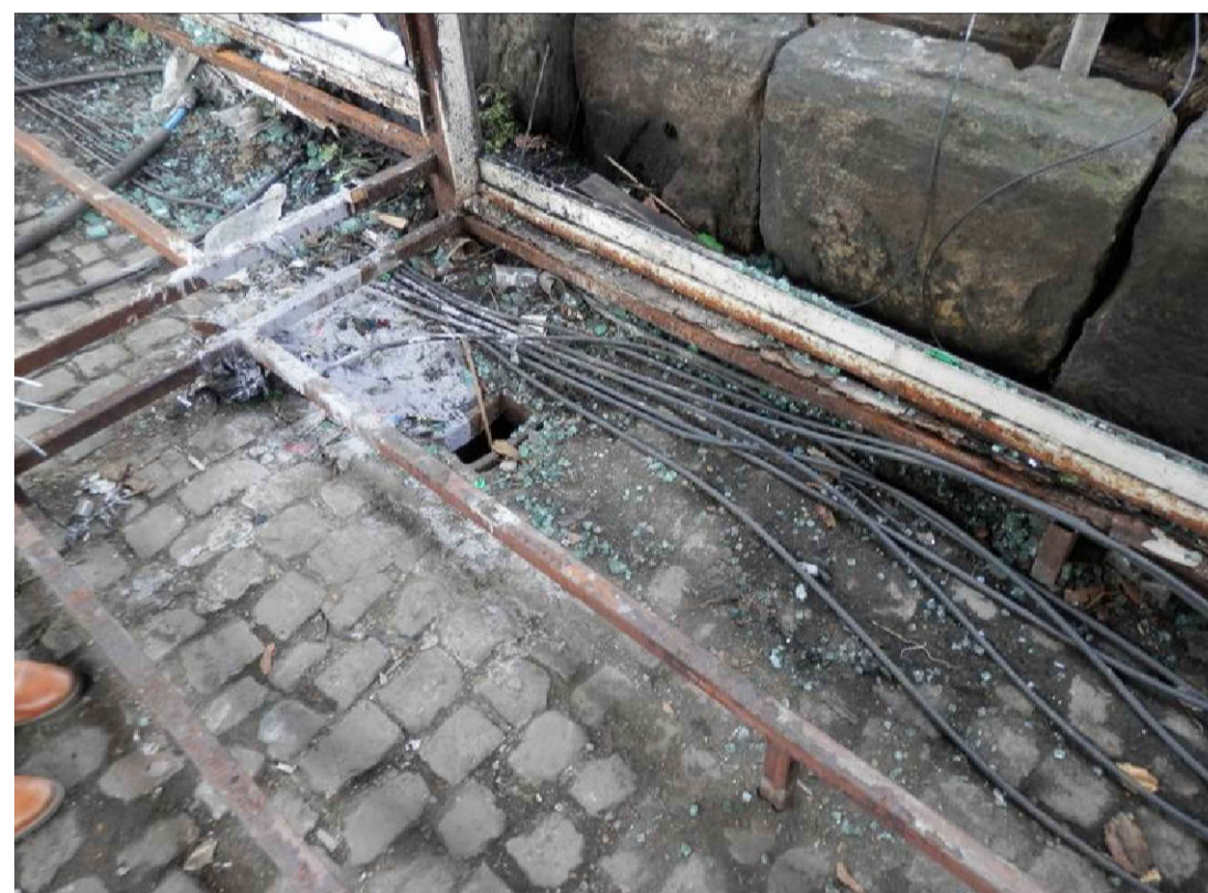
PHOTO 3 EXISTING SURFACE WATER GULLY IN COBBLED DRAINAGE CHANNEL
