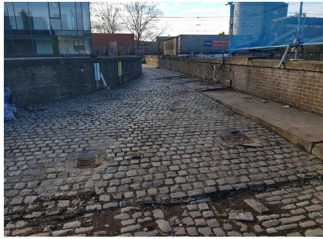
PHOTO 1 EXISTING SURFACE WATER GULLIES
