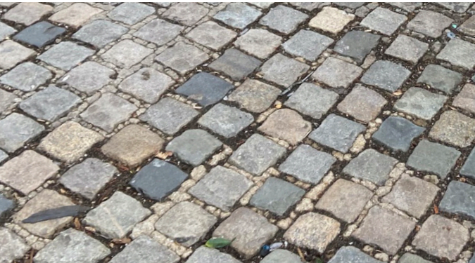
Existing flooring revealed in areas: Granite setts
