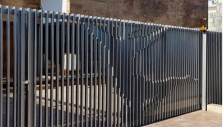
Screens: Precedent of vertical metal slats with varying depth to create an image
