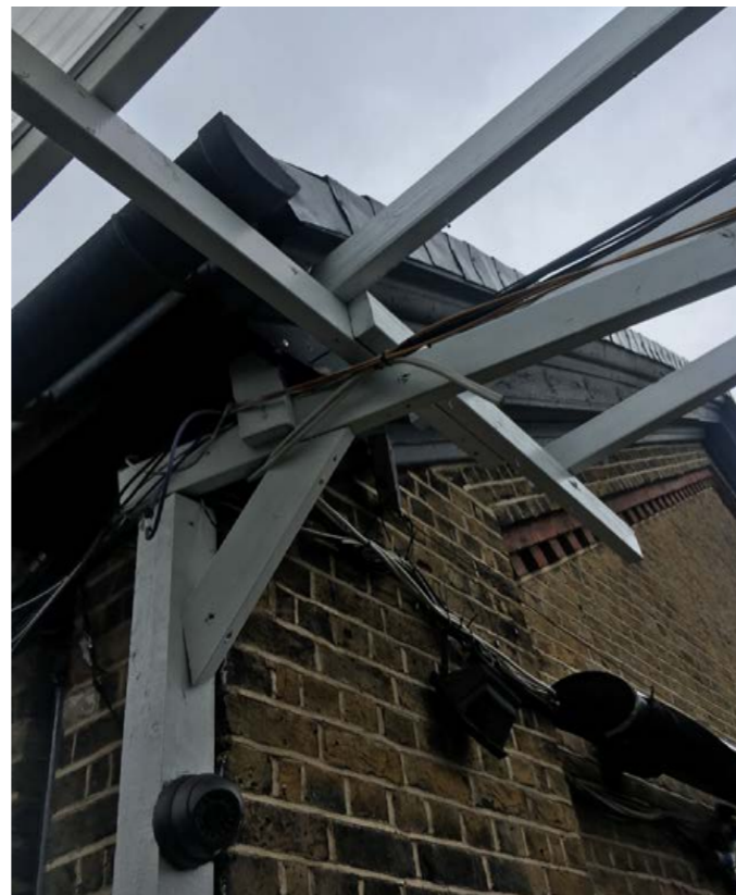
Existing Structure -to be removed.
