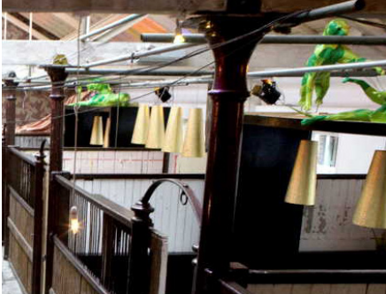
Cast Iron Columns for structure and grilles for horse stables
