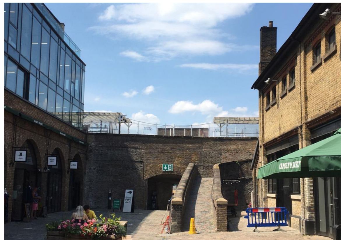
Existing view from Camden Market towards terrace at first floor level
