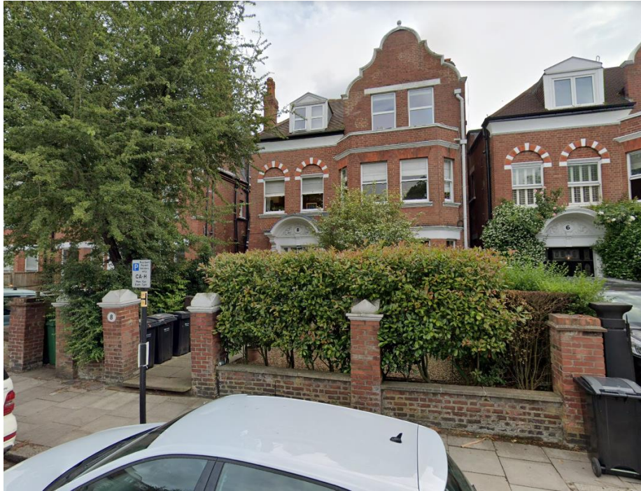
Street view of the appeal site
