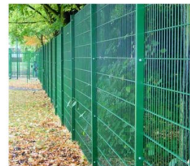
Weld mesh fencing to be used where blue lines shown to allow light into residents walkway but maintain
