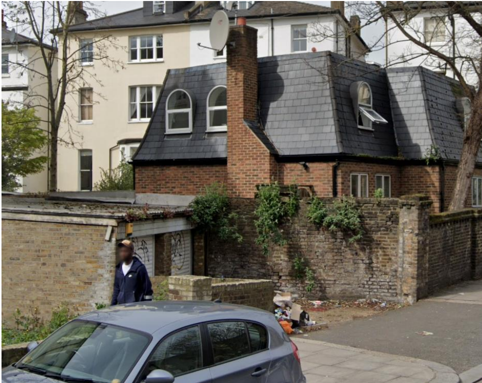
Image 4 – Priory Lodge, West elevation
