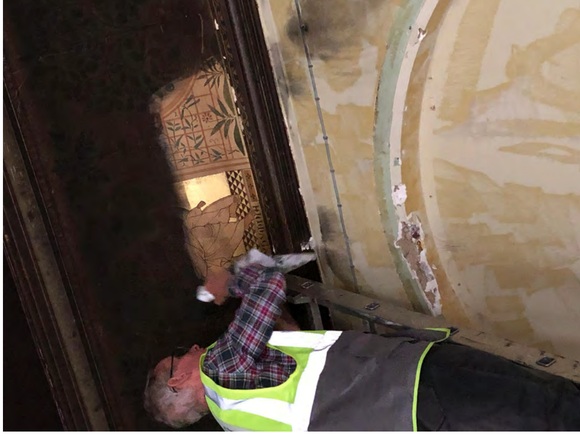
Figure 30: Initial test cleaning of the fire and smoke damaged frieze
