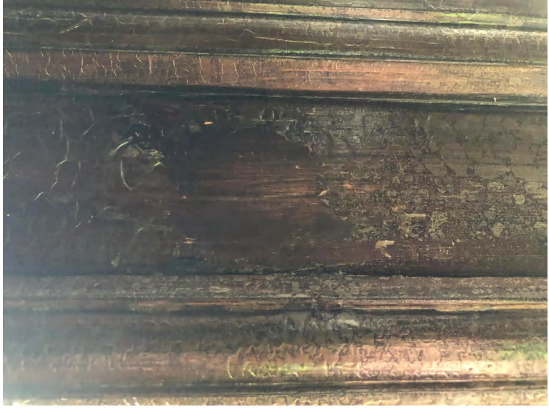
Figure 24: On closer inspection the acrylic varnish can be seen to have bubbled and readily peels away from the paint surface beneath
