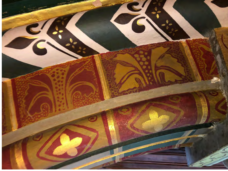
Figure 67: Current neo-gothic paint scheme in modern materials
