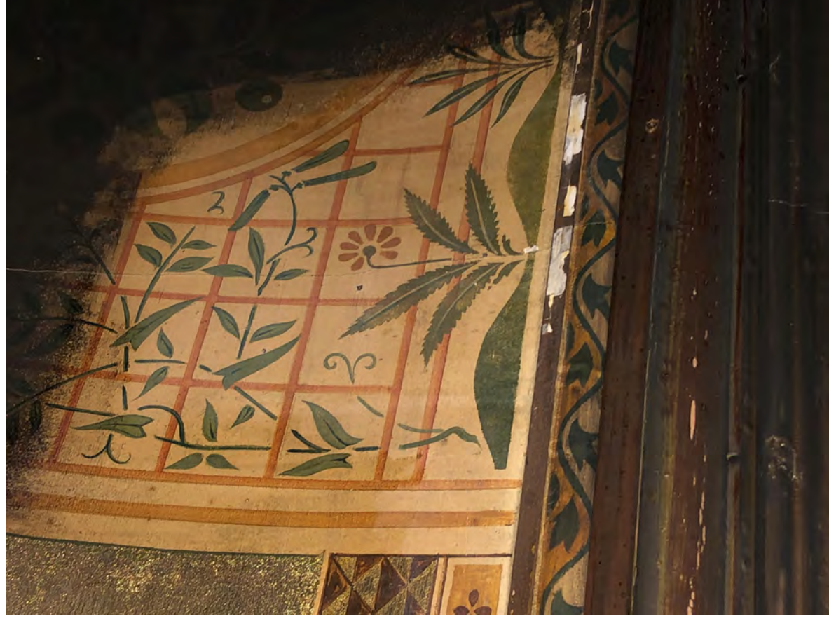
Figure 32: Detail of plain painted design area after initial clean
