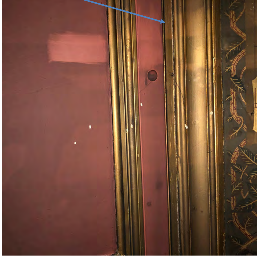
Figure 40: Room 2. Ceiling and large cove
