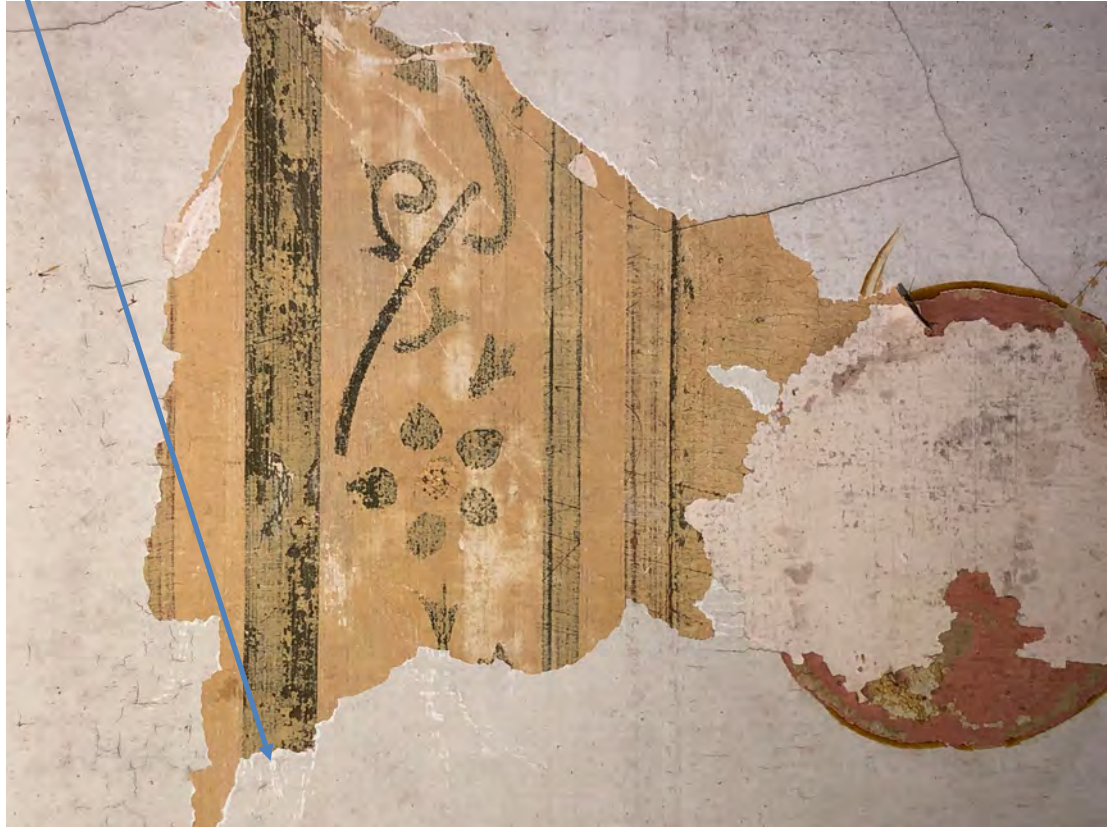
Figure 17: Room 1 Wall Face Recess Arch
