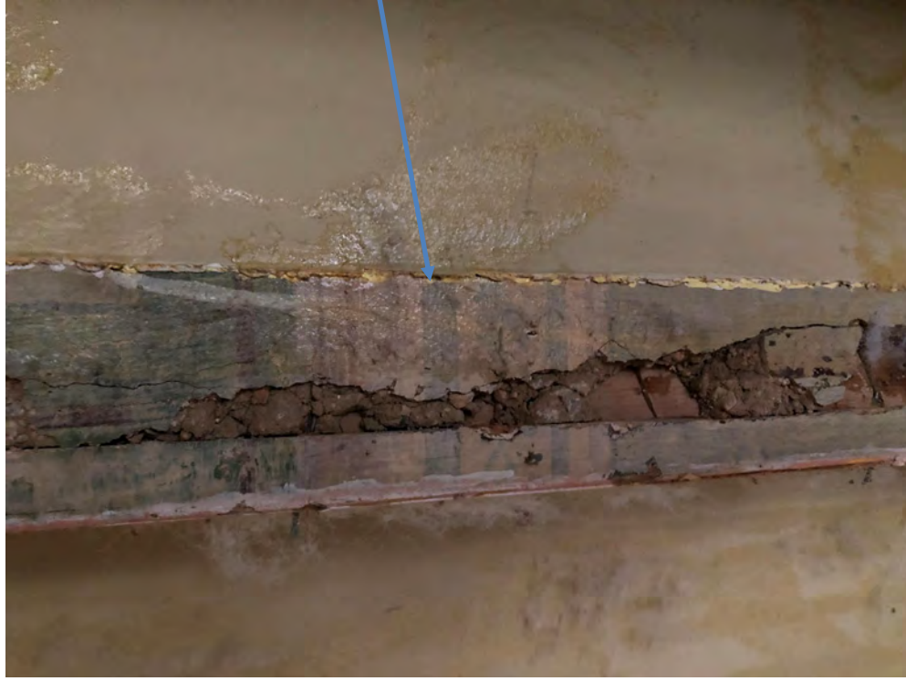
Figure 27: A scar where a later timber has been removed exposing the original stencil frieze applied to the wall faces
