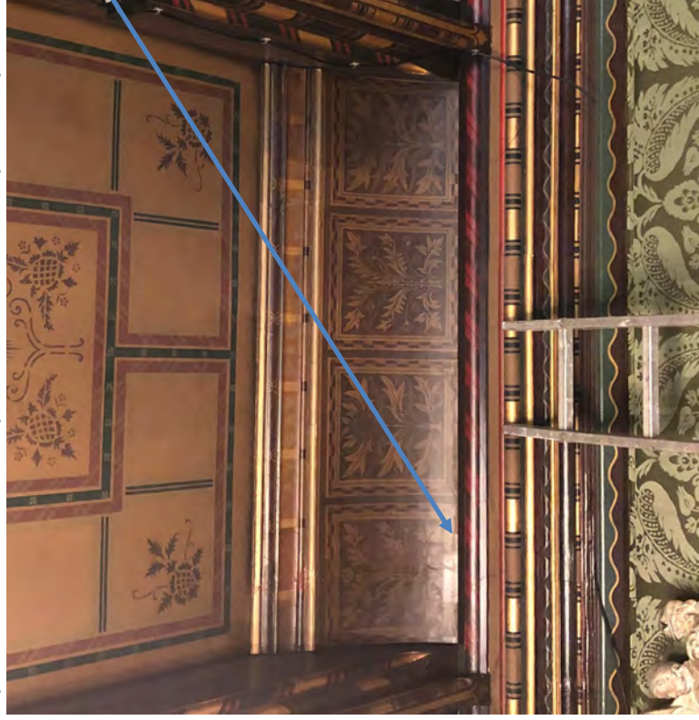
Figure 55: Room 3. Drawing Room, detail of ceiling and large cove
