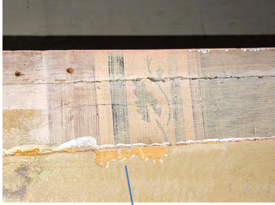
Figure 28: a clearer area of the original frieze with light overpaint
