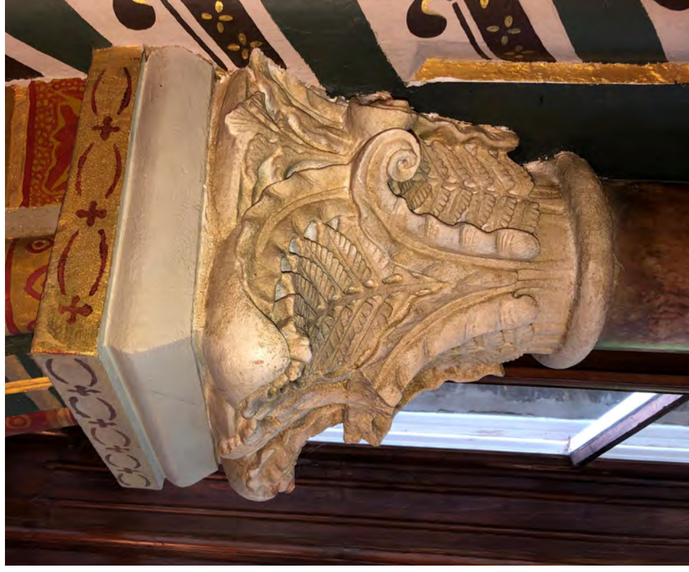
Figure 68: Modern 'stone colour' wash over the limestone capitals
