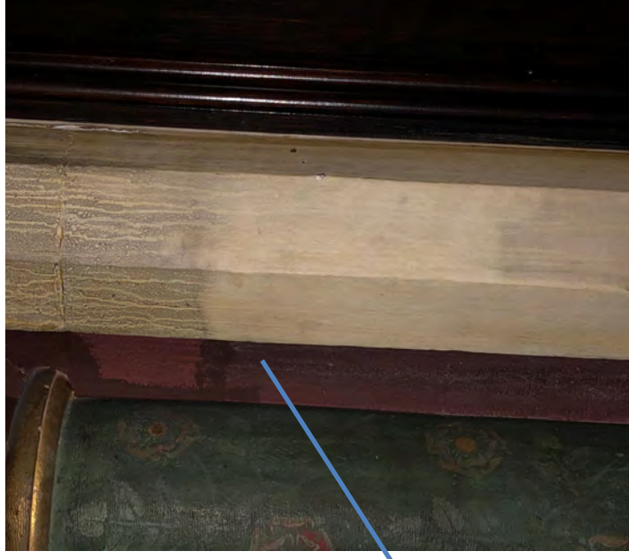
Figure 50: Room 2. Test clean to painted stone detailing
