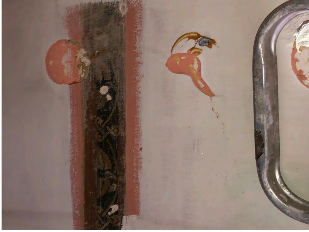
Figure 29: Area of original stencil surviving in the wall face arch recess
