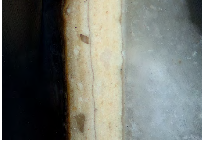
Figure 56: Room 3. Sample 6.1. Large Cove Painted Panel
