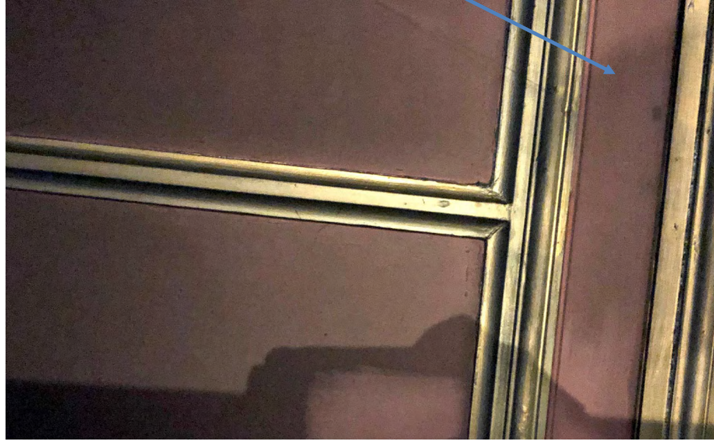
Figure 38: Room 2. Detail of ceiling panels, frames and mouldings
