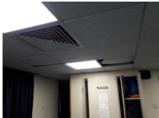
Photograph 18 – Example of a 600x600mm supply diffuser
