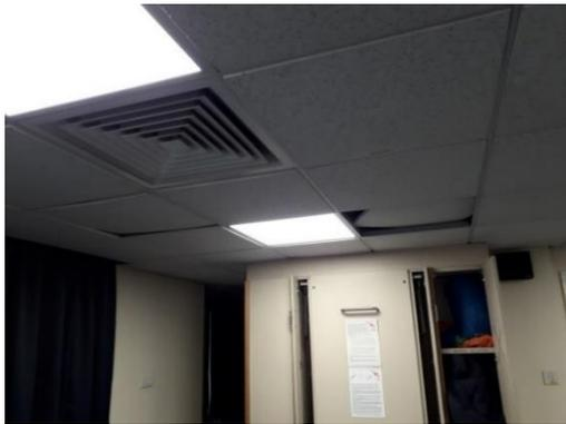
Photograph 09 – Example of a 600x600mm supply diffuser
