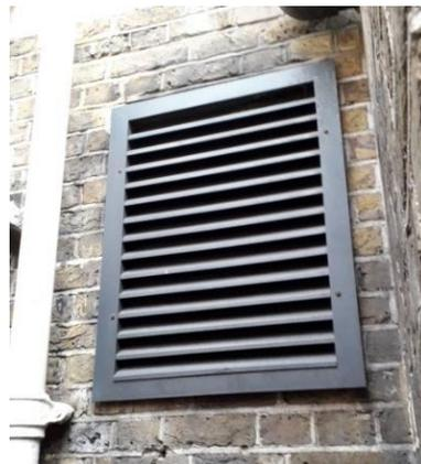
Photograph 04 – Air intake for Flue Dilution System
