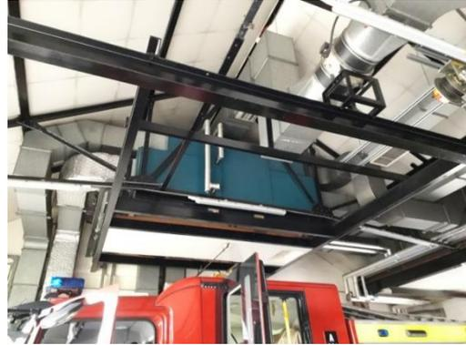
Photograph 08 – General supply and extract AHU within Appliance Bay
