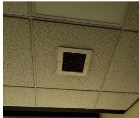
Photograph 16 – Example of a 250x250mm extract grille
