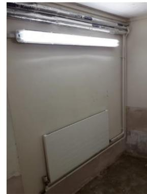
Photograph 10 – Example of SPC radiator and heating distribution pipework
