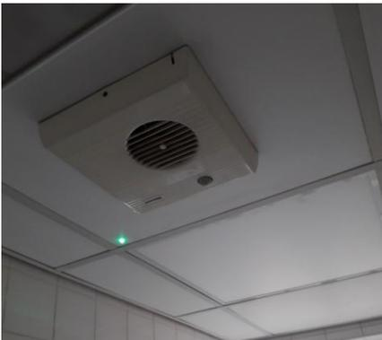
Photograph 15 – Example of a local ceiling mounted extract fan
