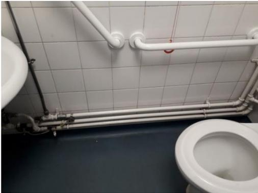
Photograph 13 – Example of domestic water services distribution pipework
