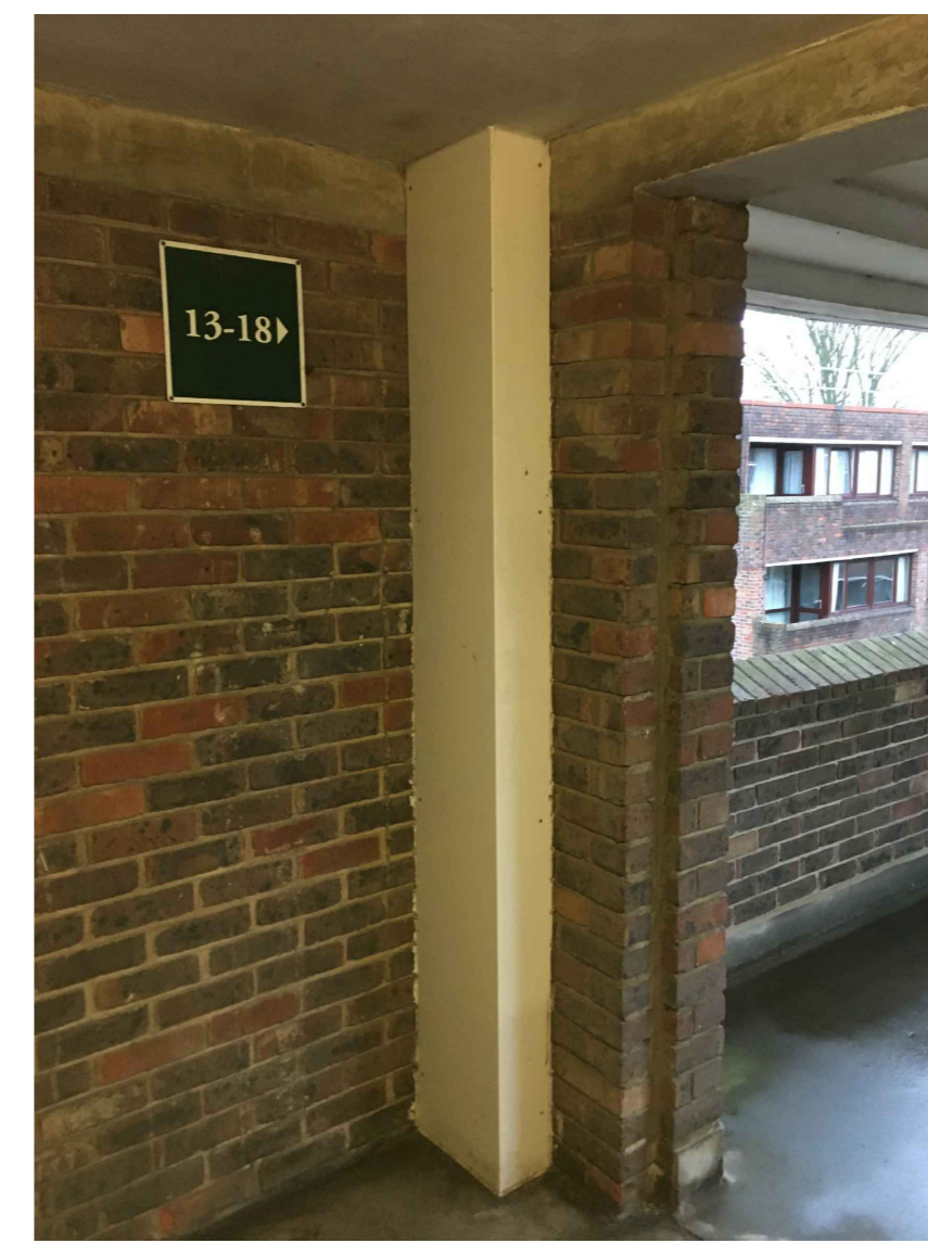
PHOTO F- 3rd floor balcony main boxing in stairwell from below.
