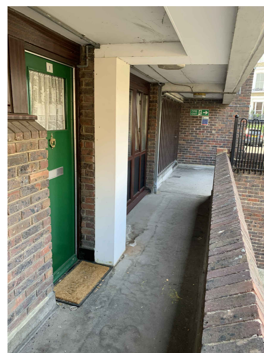
PHOTO B- 1st floor balcony showing boxing riser.
