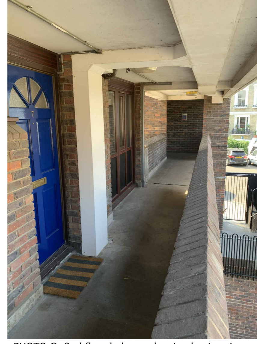
PHOTO C- 2nd floor balcony showing boxing riser and branch to stairwell.
