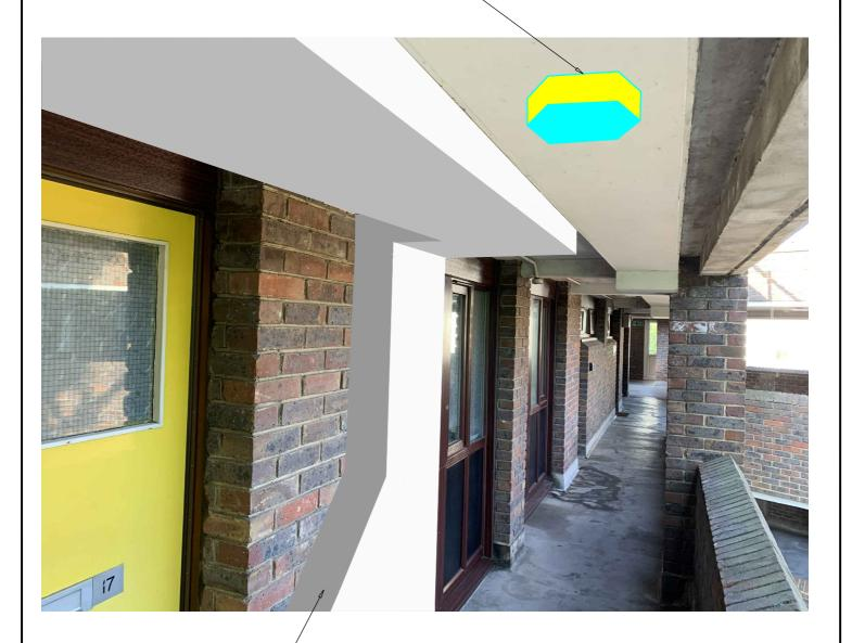
ENCLOSURE TO — ACCOMMODATE PIPEWORK OFFSET TO 1st FLOOR.
