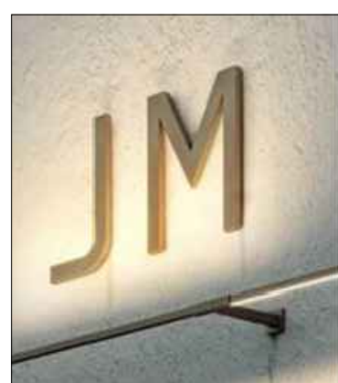
C SHAPE PROFILE (20MM X 20MM H) WITH LINEAR LED INSERT 2700° K TEMP.
