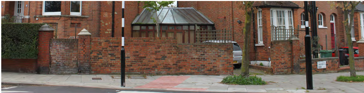
fig. 8 - Front boundary wall, cracked and varying in height.
