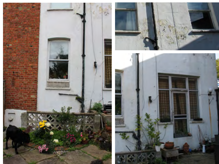
fig. 12 - Low wall to be rebuilt, damaged render and paint finish to be restored and door to be replaced.
