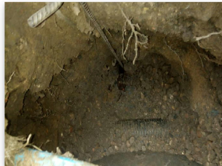
Fig 1.2: Trial Hole 1 Footing
