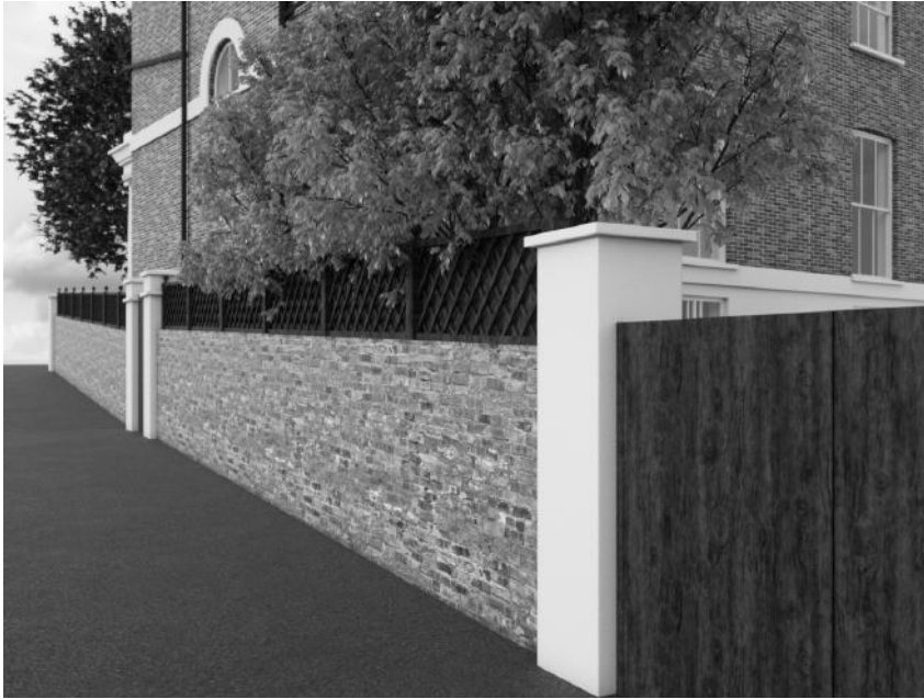
Existing View of Fellows Road Wall adjacent to the garden gate. (summer)
