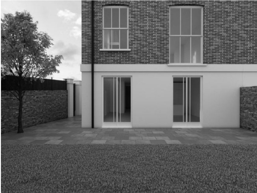
Existing Rear View from 1 Steele's Road
