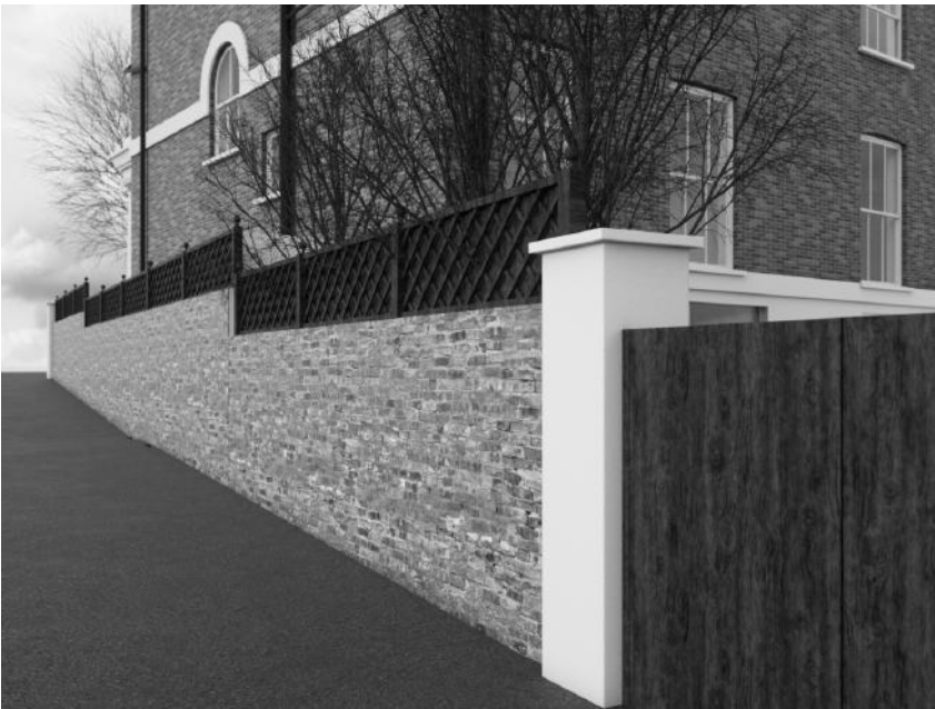
View of Fellows Road Wall adjacent to the garden gate. (winter)
