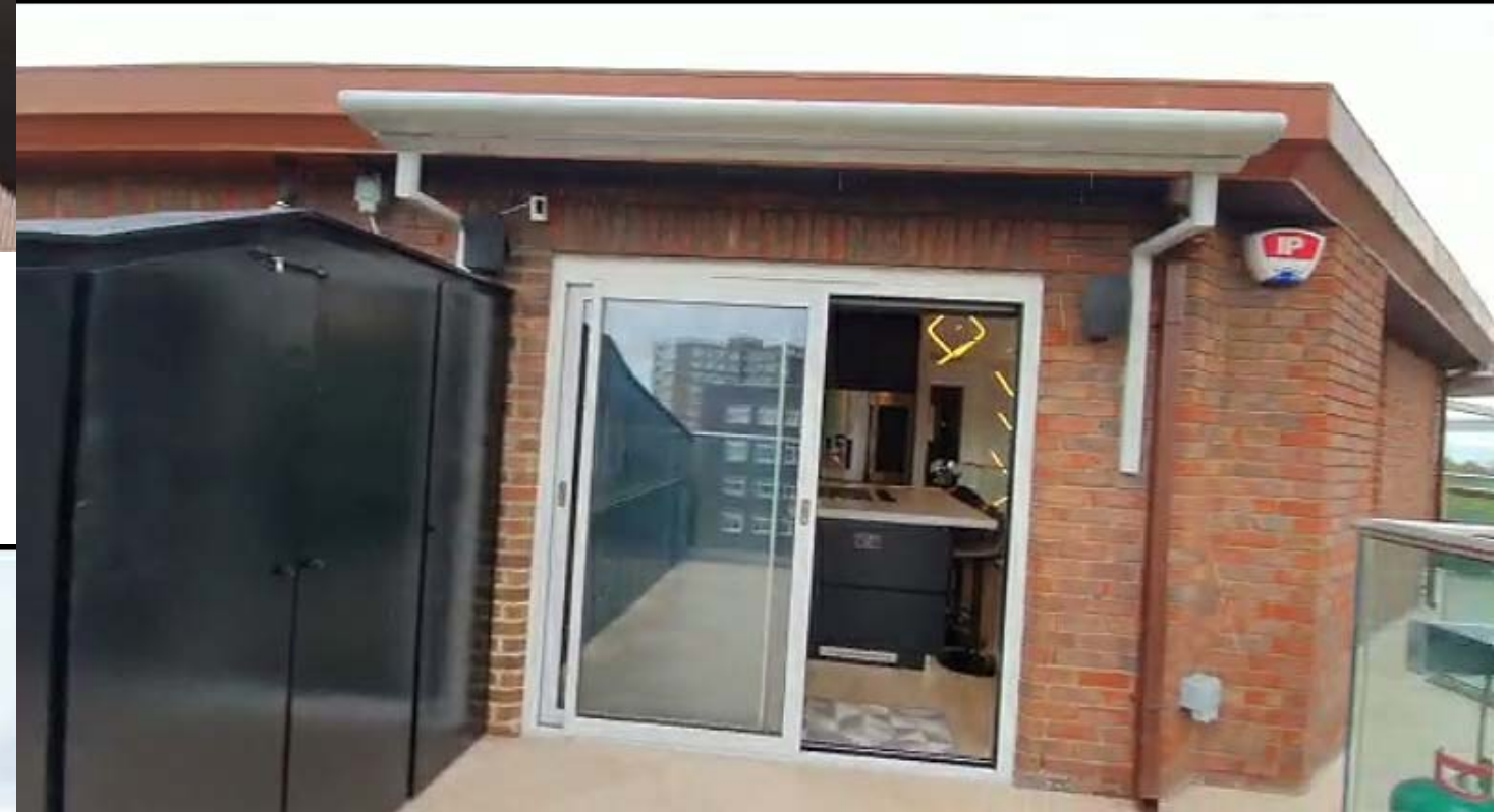
VIEW FROM TERRACE TOWARDS FLAT
