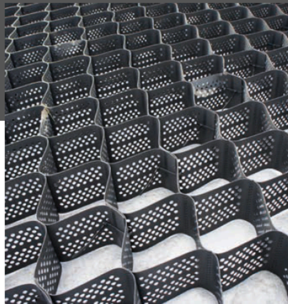
ProtectaWeb™ TRP System being pegged out
