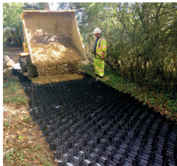
ProtectaWeb™ TRP System being infilled with stone
