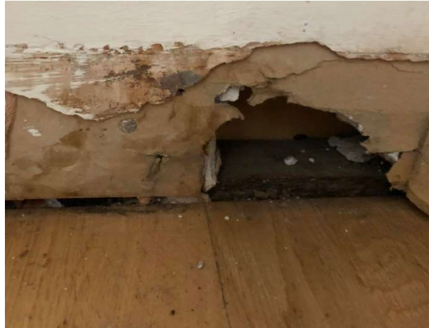
Base of stud wall showing plasterboard construction
