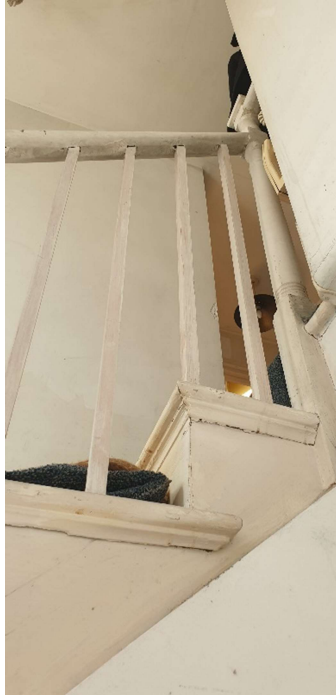
Existing staircase string, balustrade and handrail detail
