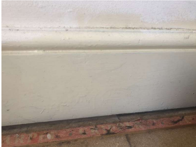
Existing skirtings to external walls & party walls
