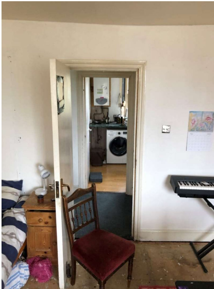
Intermediate stud wall with bullnosed skirtings on chipboard flooring
