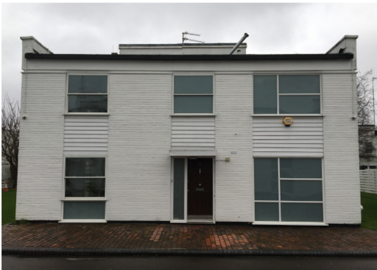
2. Existing front elevation (viewed from pavement opposite the site)
