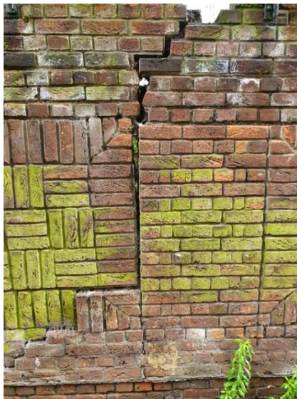
Figures 4.2 Damage to the garage structure
