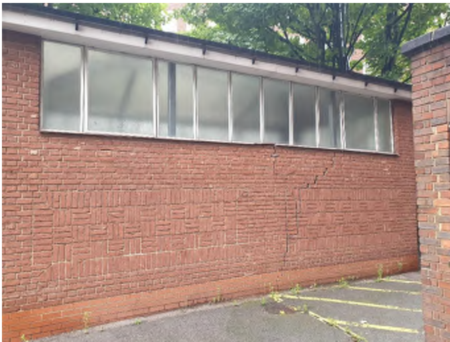
Fig. 1 Damage to the retaining wall
