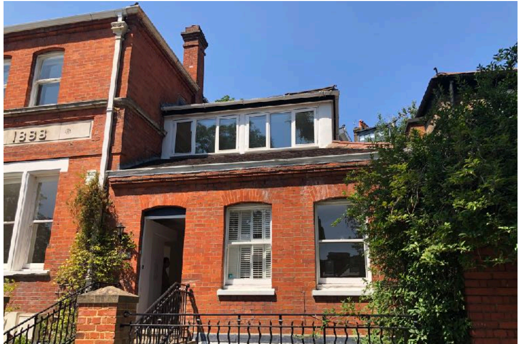
Lower side wing with strip of EMJA casement joinery windows to first floor bedroom
