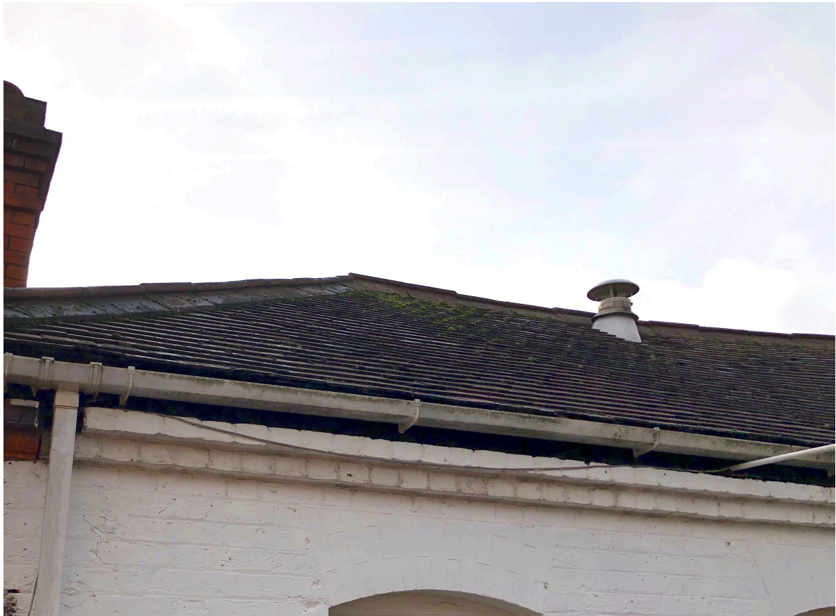
part rear roof slope with existing gas flue terminal
