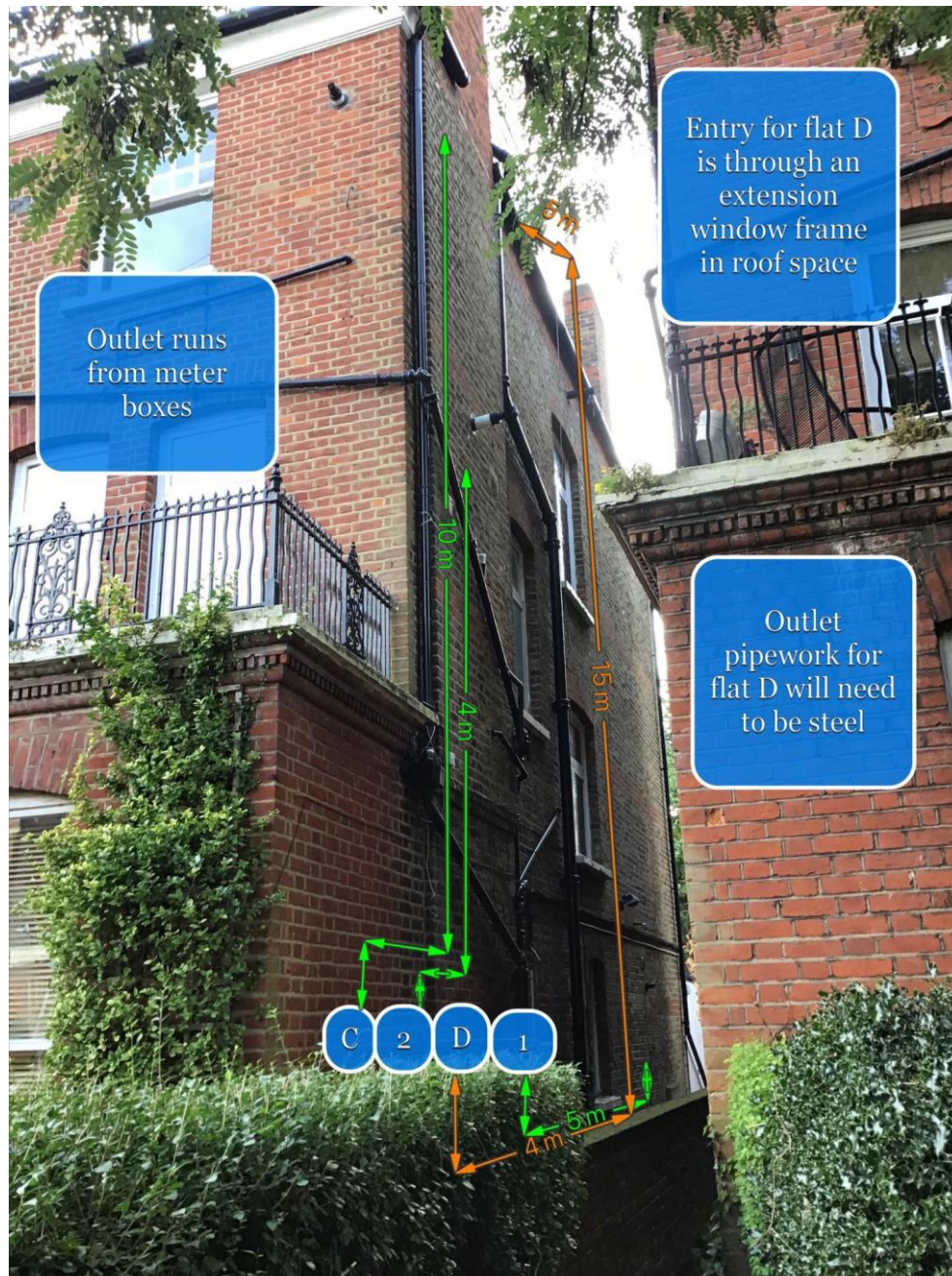
Plate 1 - Indicative image illustrating the positioning of the new gas pipe apparatus on the west (side) facing elevation of 59 Compayne Gardens.
