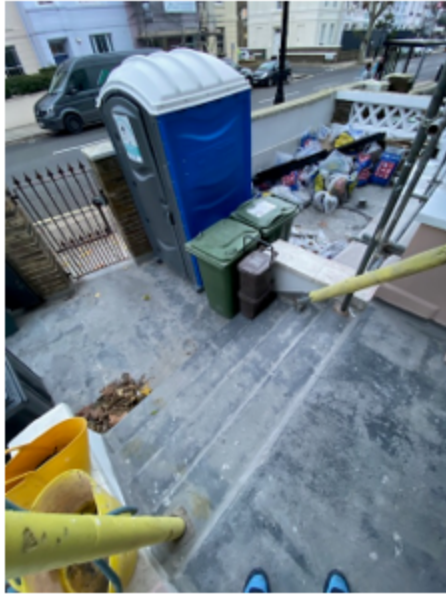
Existing front garden and steps:
