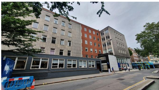
Photograph 1 Southern aspect of building B1 showing main frontage.
