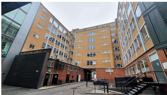
Photograph 4 Northern aspect of B1 showing hardstanding courtyard and Cypress Place alleyway running underneath B1.
