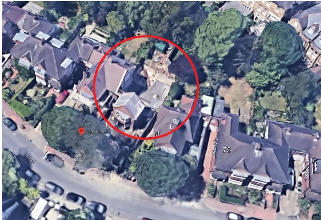
Figure 17 – Satellite view of demolition works as part of basement build at no.77 Lawn Road
