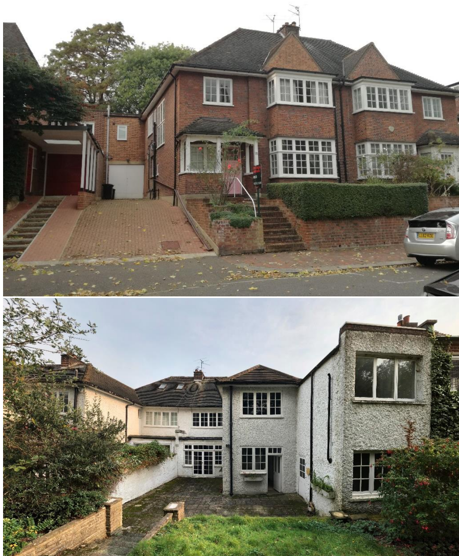
Figure 2 – Front and rear photographs of 75 Lawn Road
