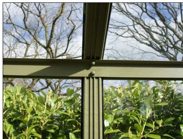
Close up view of the glazing bar with external capping profile (left) and frame connection forming the eaves.
