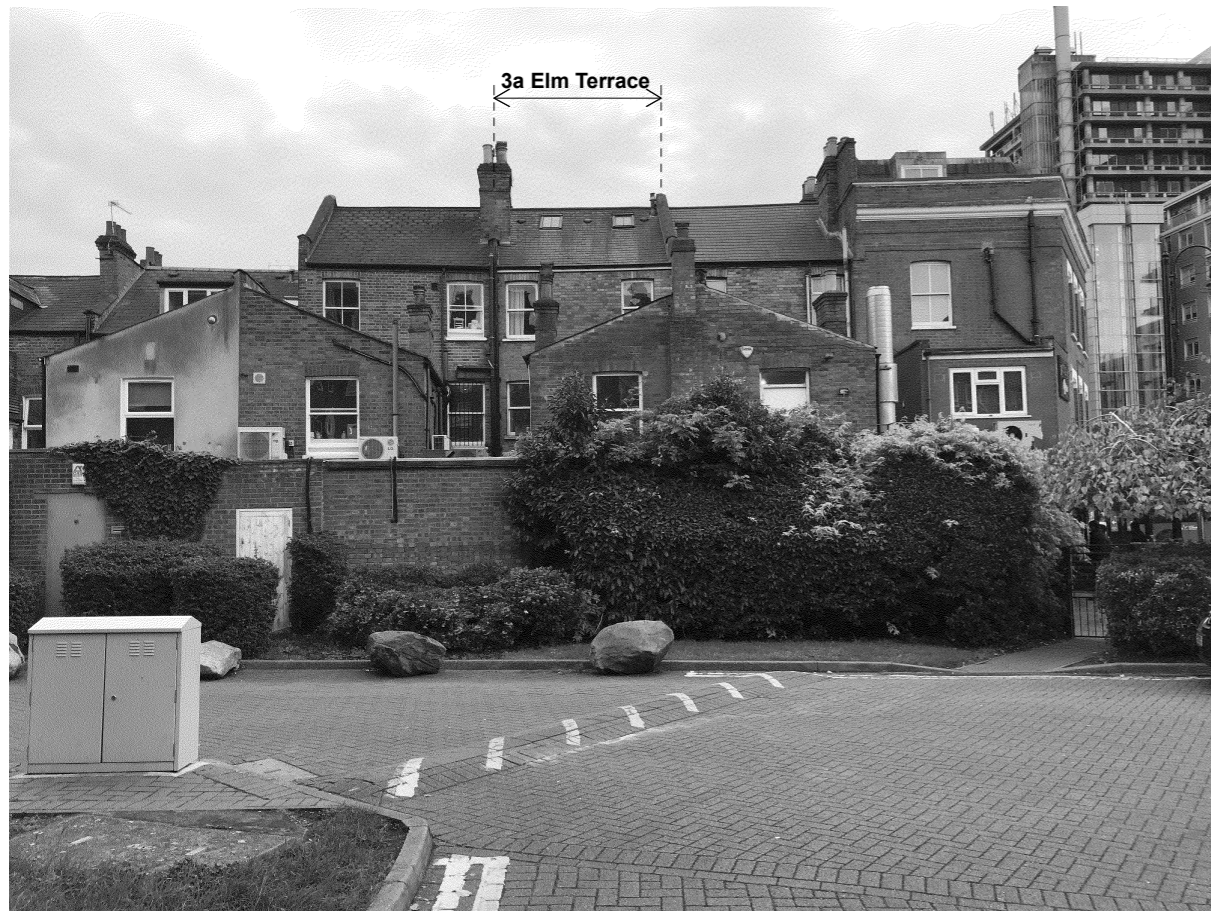
REAR ELEVATION from South End Close
