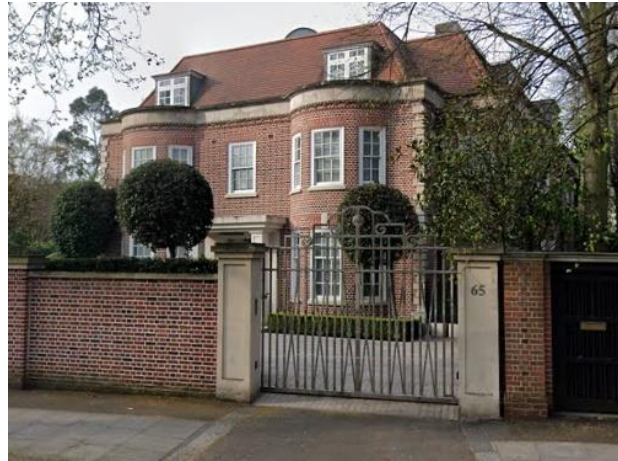
Figure 2 – Neighbouring property, 67 Avenue Road
