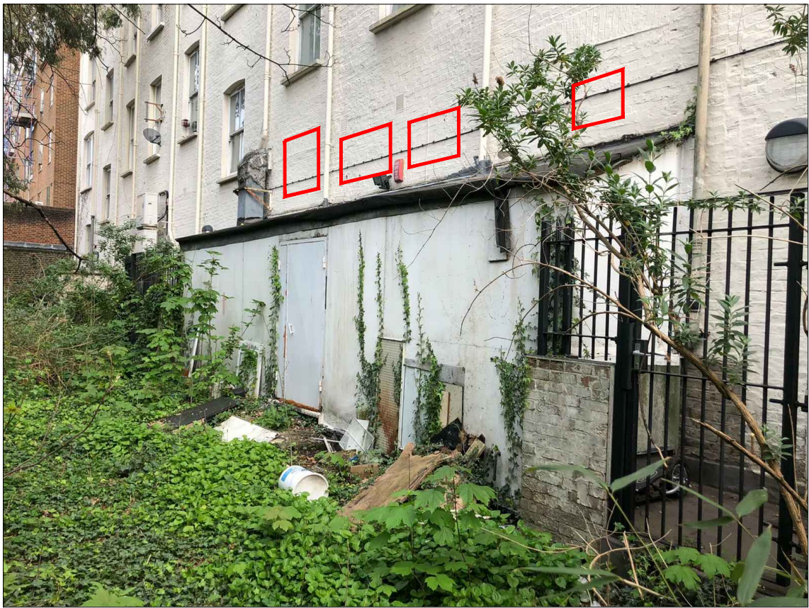
EXISTING SITE PHOTO
