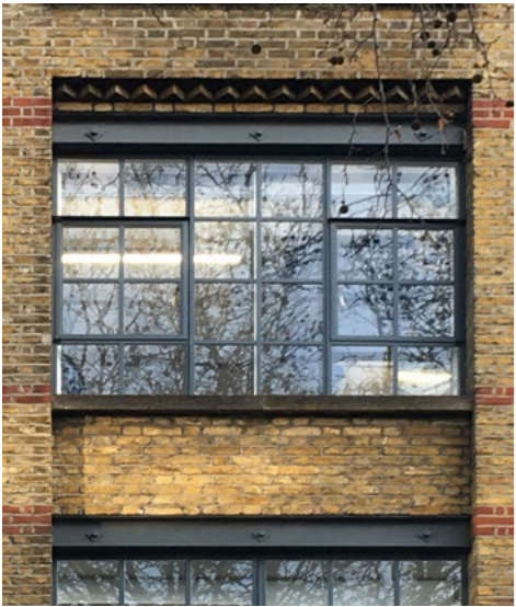
Rotated bricks lintel detail in warehouse in Stanhope Street
