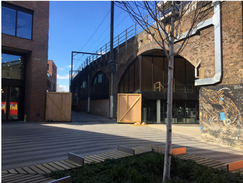
Fig 14. View of Arch N7 and site approach
