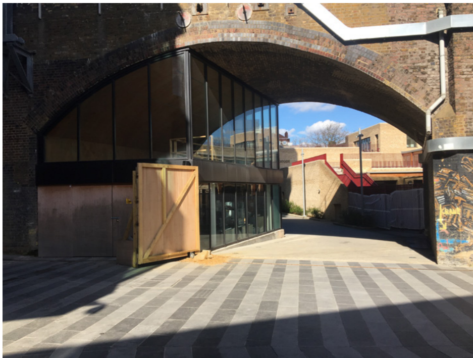
Fig 15. View of Arch N7 and route north through to Harley Road
