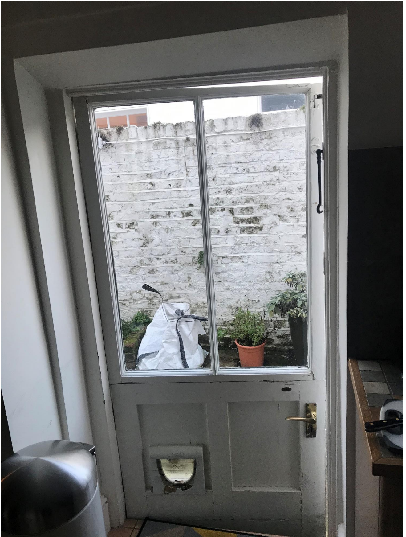
Kitchen door as existing. The uneven architraves suggest that this has been altered in the past.
