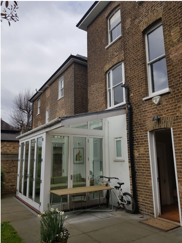
Existing rear conservatory
