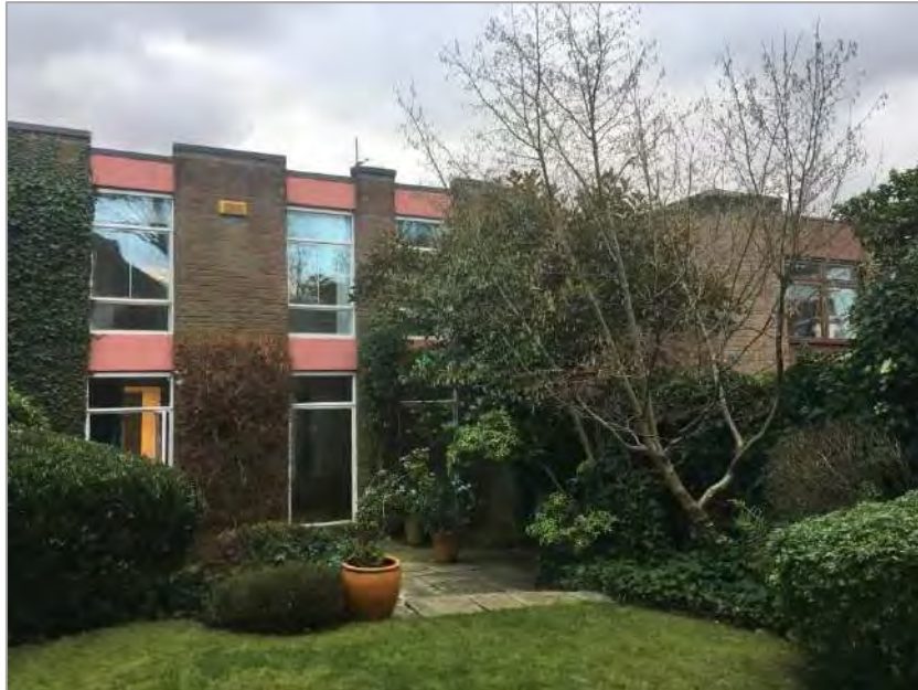
Image 9. Rear (north face) of the house.
