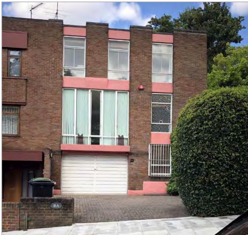
Image 2. No 18A Frognal Gardens (south frontage).
