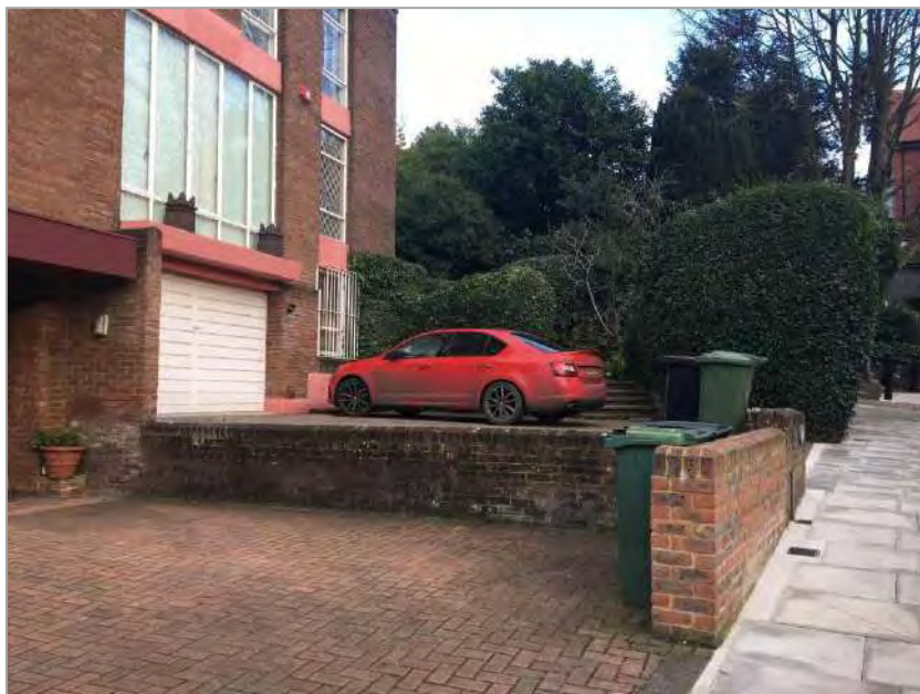
Image 4. Height differential between Nos. 18B (left) and 18A.
