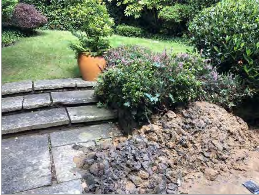
Image 11. Spoil from TP1 (patio).
