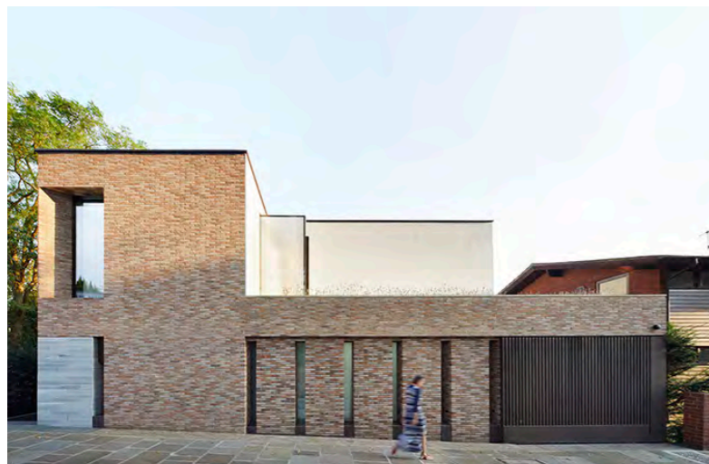
Admiral's Walk by Stanton Williams shows a non-traditional approach to brick architecture
