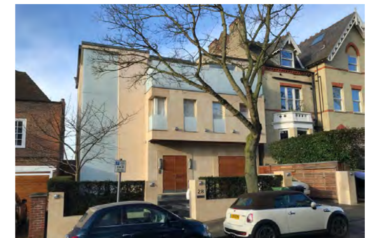
No 28 Ellerdale Road
