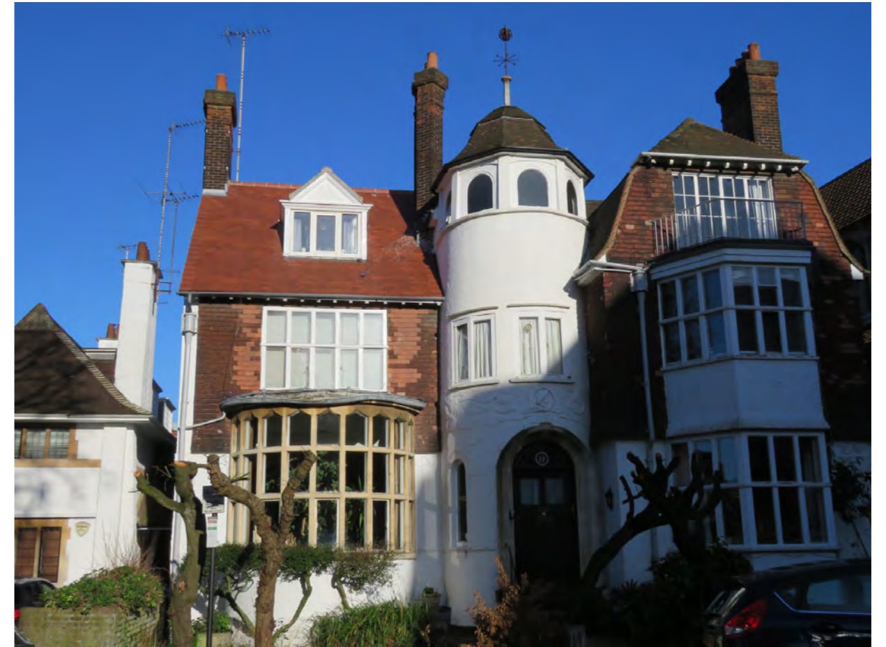
No. 14 Kidderpore Avenue shows a range of building materials, including terracotta tiling
