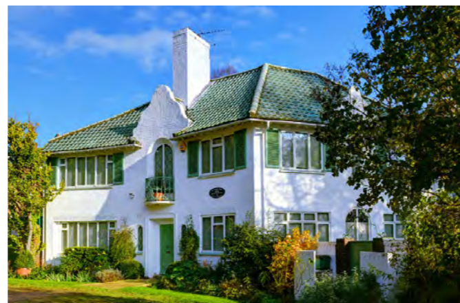
The green tiles of the 20 Frognal Way has a strong presence in the conservation area.
