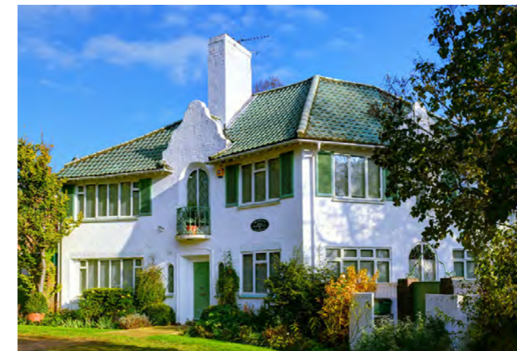
20 Frognal Way has green roof tiles and details
