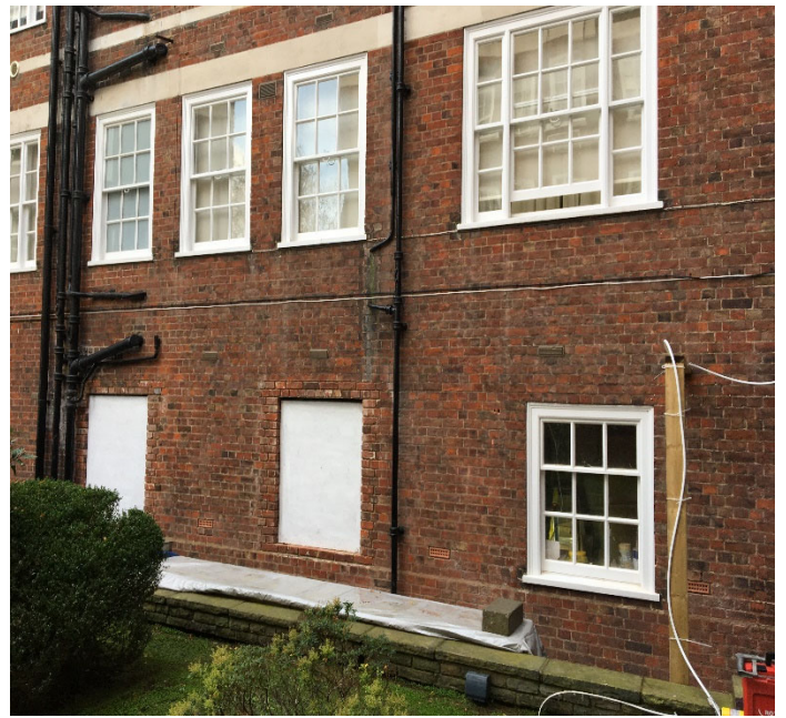
Image 4 – Existing 3 over 6 window to North elevation
