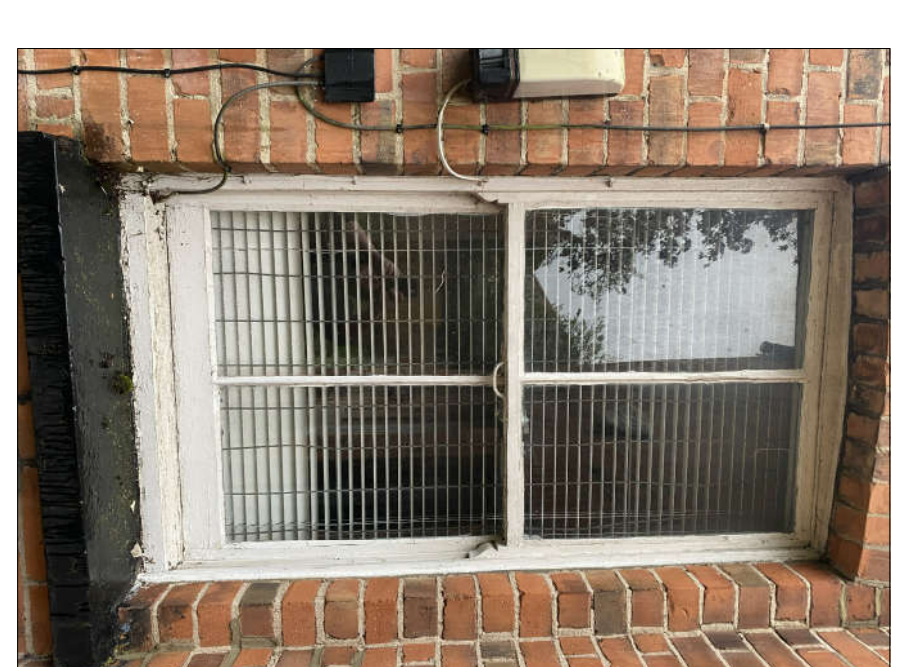
Typical Existing Sash Window
