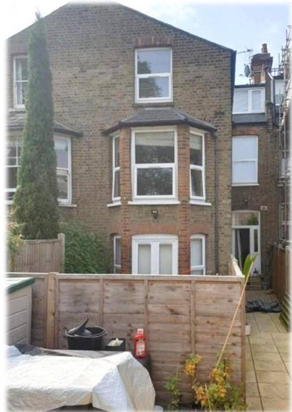
REAR ELEVATION AND PATIO AREA, SHOWING THE INTERNAL DIVISION OF THE AREA
