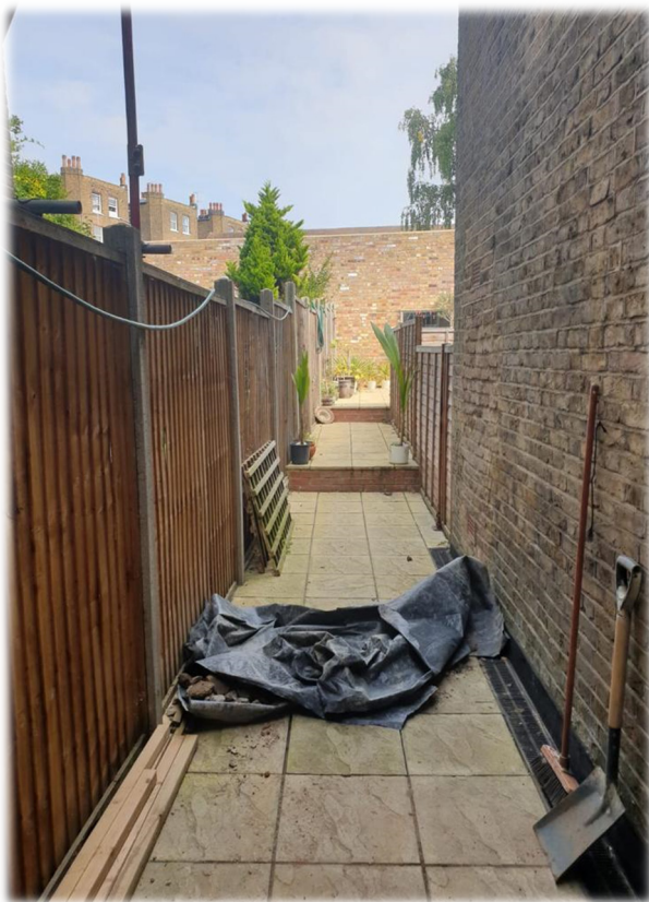
VIEW TOWARDS THE REAR OF THE SITE, SHOWING THE PARTIAL RETAINING WALL TO THE PLAYING FIELDS
